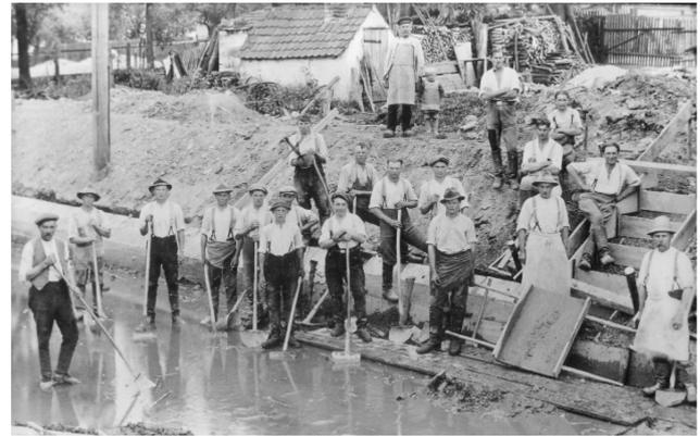
**Figure 7.** Widening of the Ach River at Grabmühle in 1927 as part of the drainage measures. The Ach River is a left tributary of the Paar River (photograph: Archiv Stiftung Donaumoos, Inv. No. 1901).
